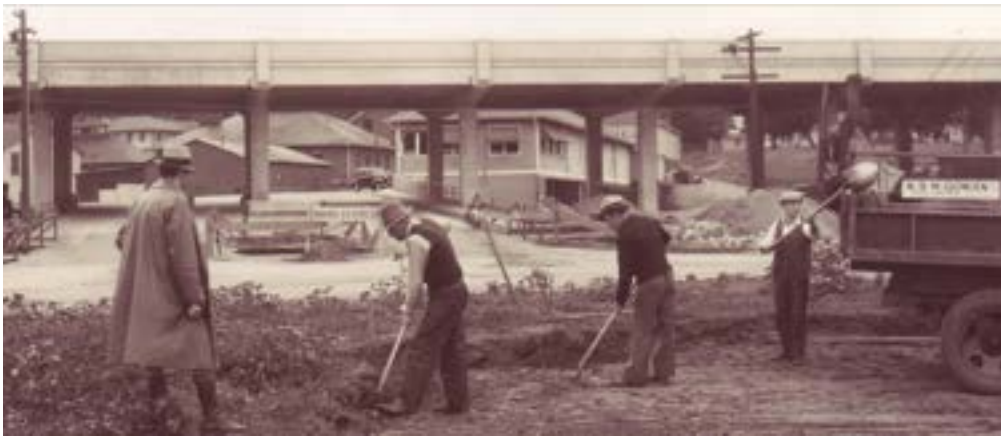
Building 201 in 1937 (center — the building with awnings) after it was relocated for the construction of Doyle Drive. Courtesy Presidio Trust.
