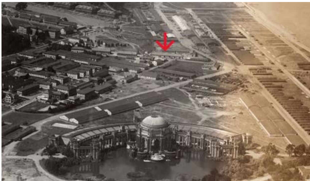
The red arrow points to Building 201 in its original location, circa 1922. Courtesy Presidio Trust.
